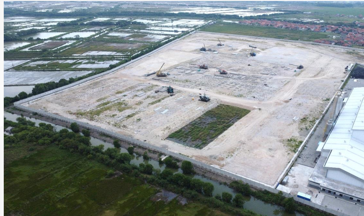
1 st April 2024 - Avian Brands' third factory construction in Cirebon, West Java
